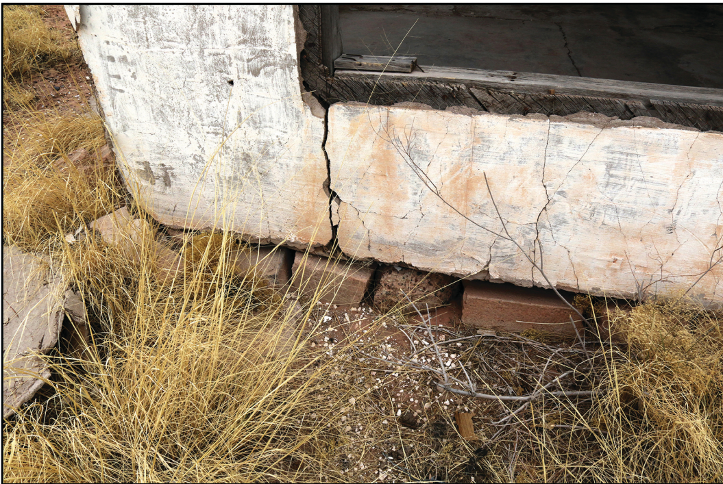
Southeast corner. View toward the east wall.
