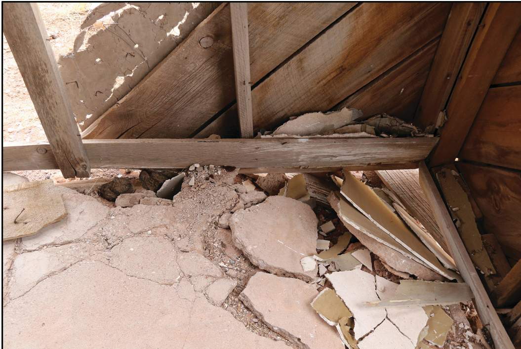
Interior view of the southwest corner.
