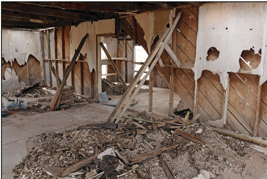
Interior view in present condition looking toward the northwest.
