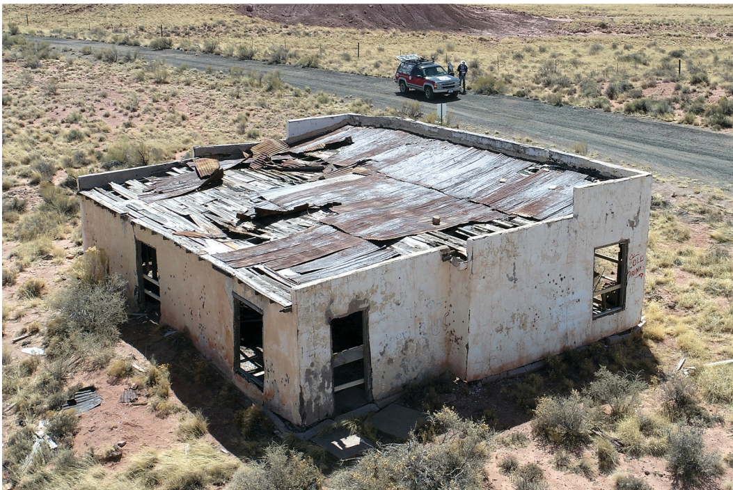
Eastward view of overall structure.
