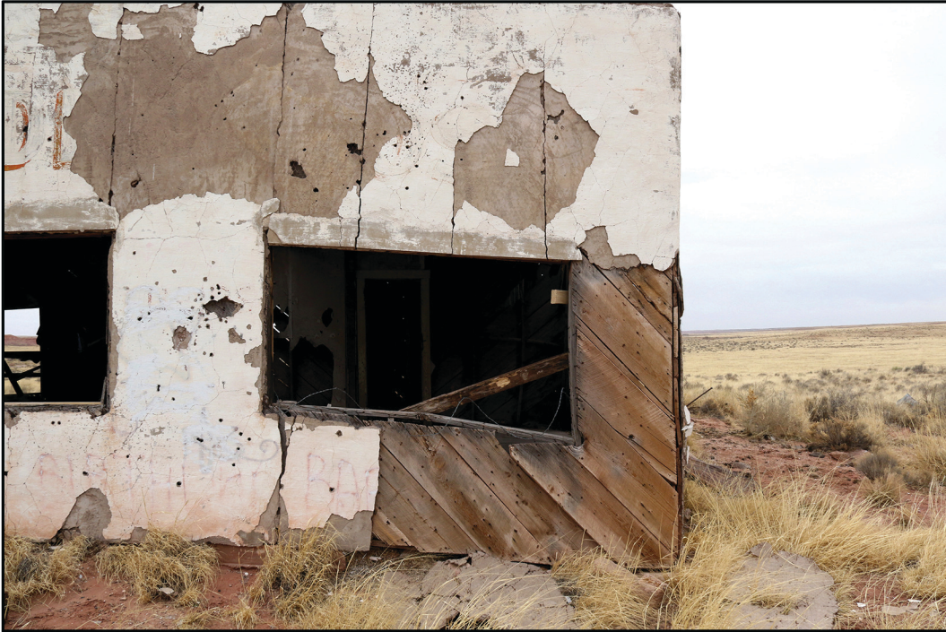
Southeast corner of the trading post. View toward front wall.
