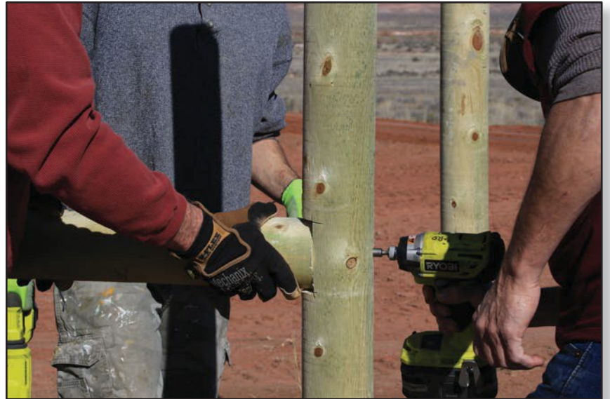
Crew members assemble corner posts.
