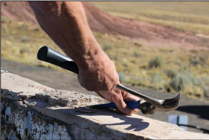
The parapet walls required labor intensive prep for stucco repair and capping.
