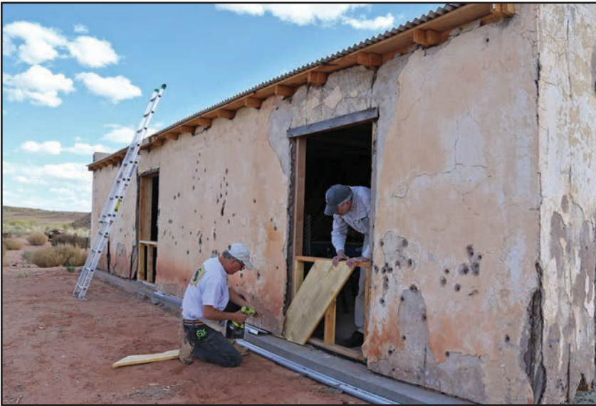
Sheathing is replaced under the rear windows.
