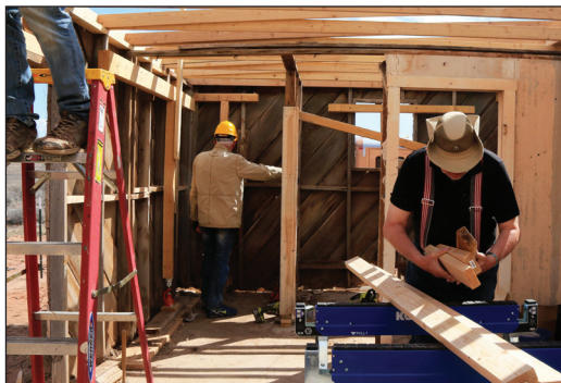
Jack posts in position in the NE corner.
