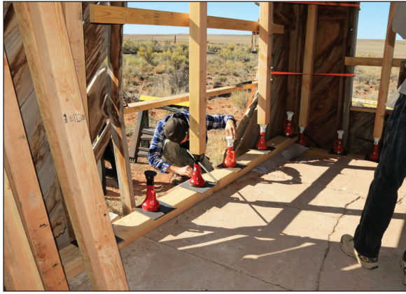
Preparing jack posts for lifting the SW corner.
