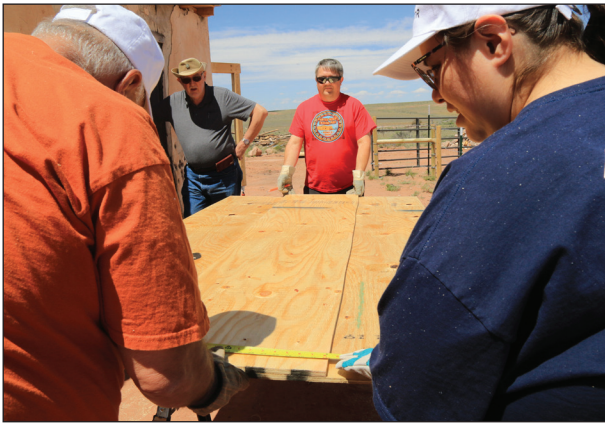
Workers cutting plywood for concrete forms.
