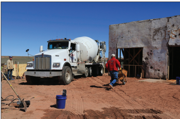
The first concrete truck arrived at 9:00 a.m., Tuesday, May 28, 2019.
