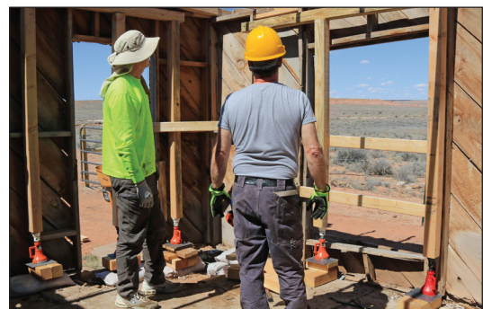
Jacks and jack posts in the NW corner.
