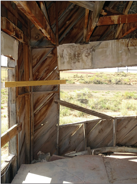
View of SE corner (camera facing south). NPS
