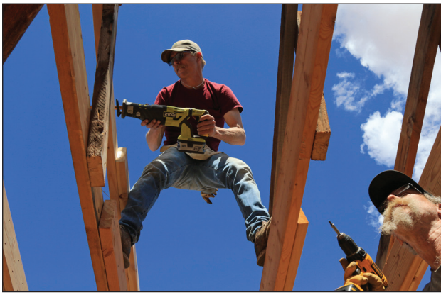
Installation of new rafters, incorporating original diagonal braces.
