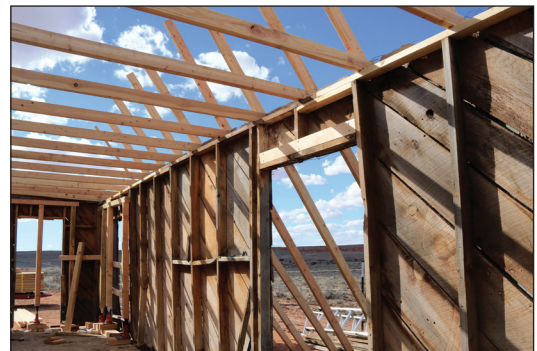
Installing new ceiling joists in rear room.
