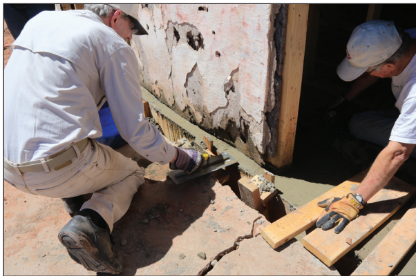
Finishing touches are given to the concrete as it hardens.
