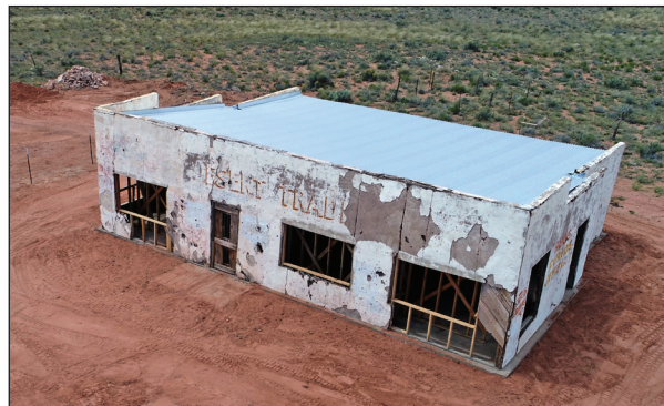
Finished roof. Photo taken after completion of Phase III.
