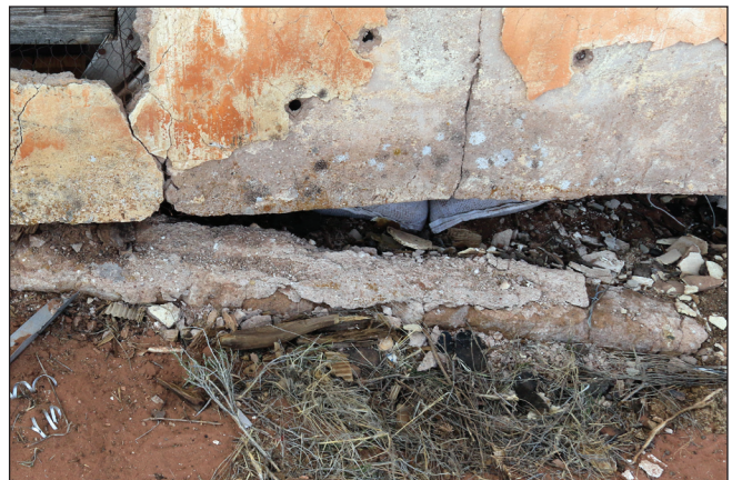
Collapsed foundation.
