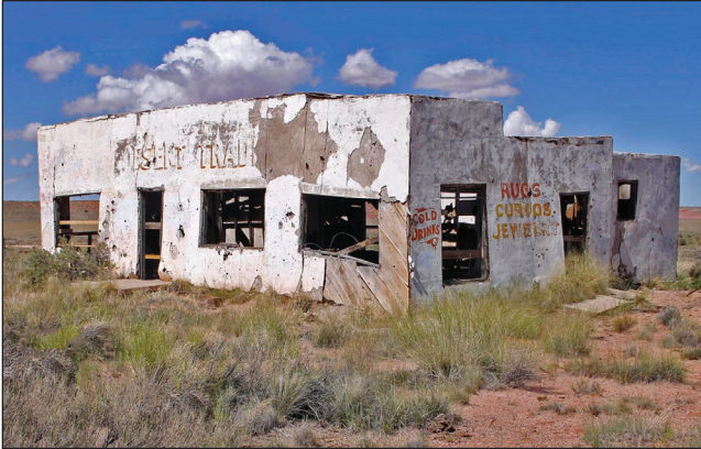
View of front and east walls. Lisa Drewitz
