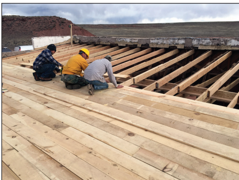
Views of the new roof structure and decking (above and left), and the roof as seen from inside the rear room.
