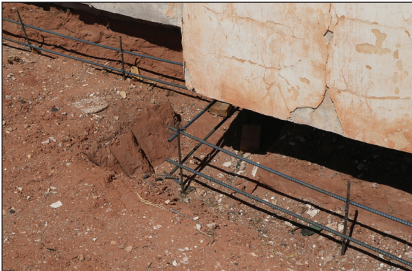
Rebar used was 1/2" in diameter.
