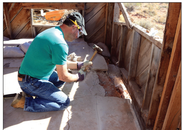
Removing unsupported concrete to allow space for sandbags and timbers.
