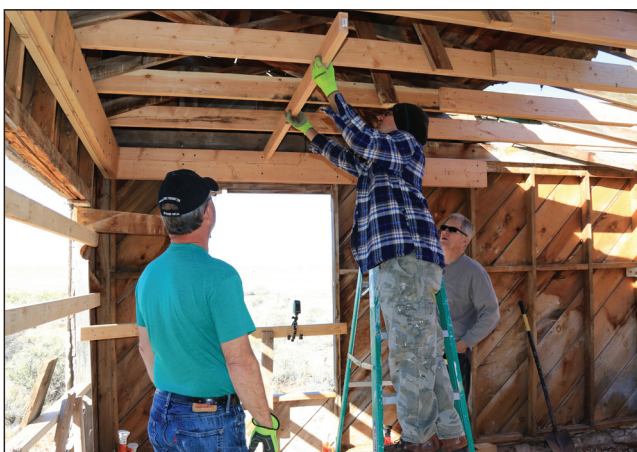
View of replacement joists and timber beams bolted to walls.
