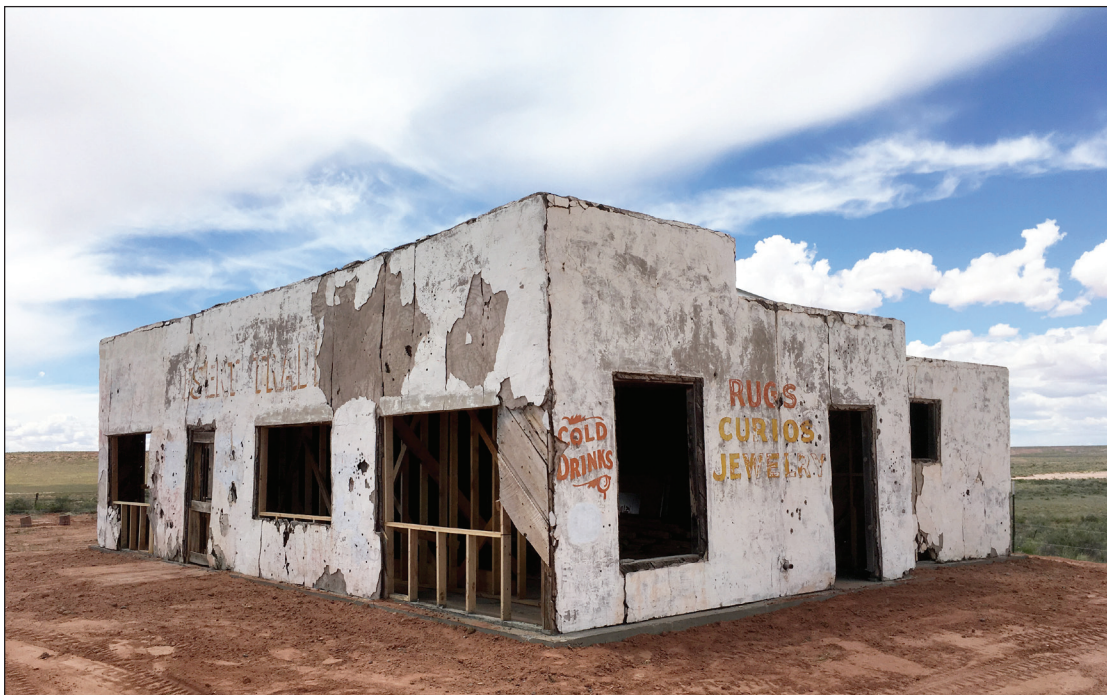
The new foundation after backfilling.
