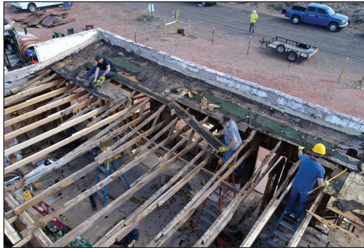
Removal of existing roofing.
