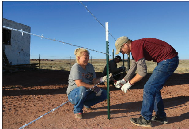
Installing the fence.
