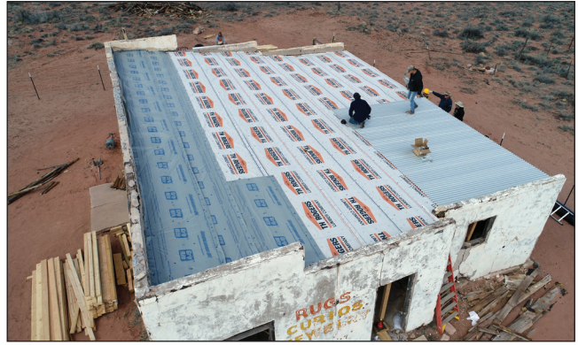
Corrugated Galvalume was used for the sheet metal.
