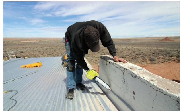
Silicone sealant being applied to the end-wall flashing.
