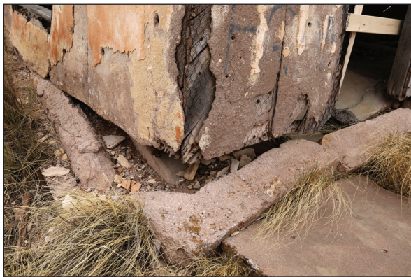
Foundation at NW corner.
