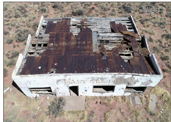
Condition of roof.
