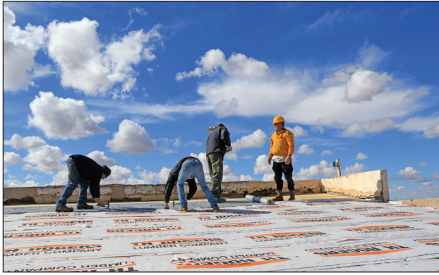
Synthetic underlayment being applied over the roof decking.
