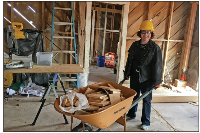
Continual clean-up by volunteers helped keep work spaces unencumbered.
