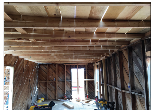
Views of the new roof structure and decking (above and left), and the roof as seen from inside the rear room.
