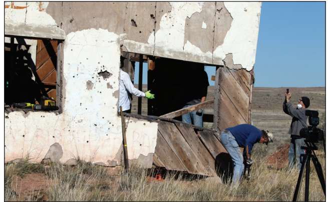
East end of front wall.
