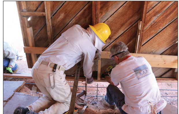
Securing new sill plate to a sistered wall stud.
