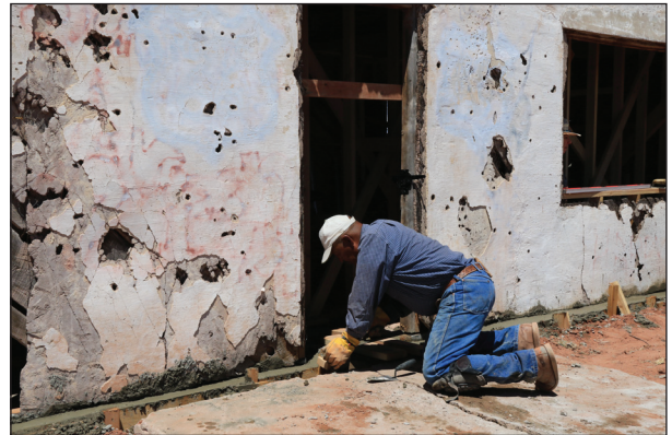
The foundation is trowelled smooth as it begins to set up.
