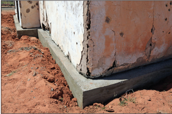
South view from NE corner following removal of concrete forms.
